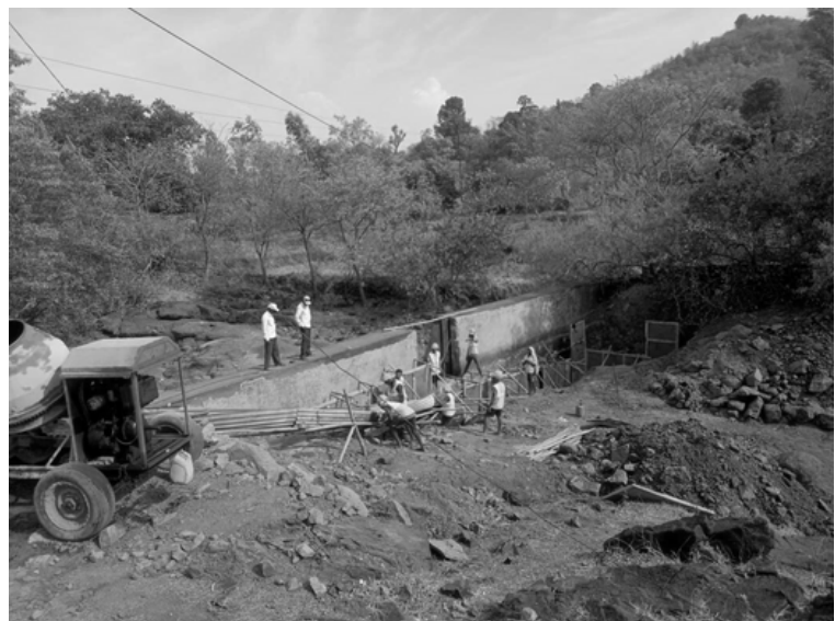
Dhanushi Check Dam repair
