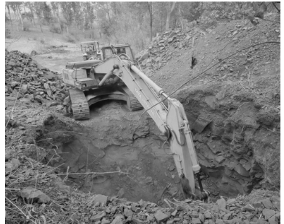
Borshet Open Well construction
