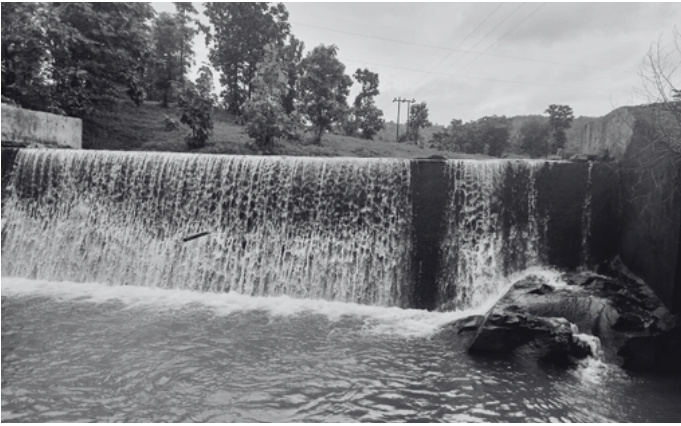
Khandipada Check Dam repair
