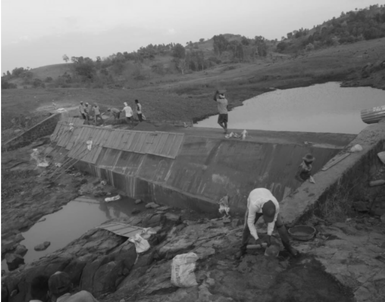
Sakhri Check Dam repair
